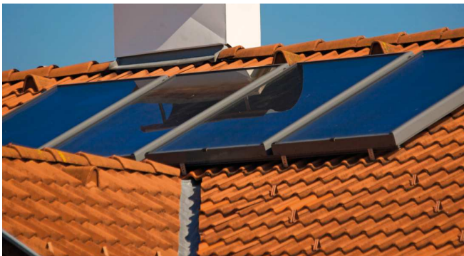
Installation on the roof
