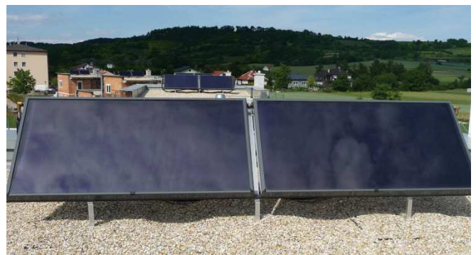
Installation on the roof – horizontal
