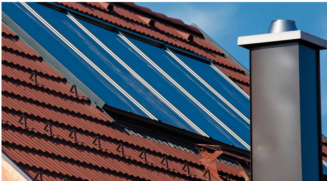
Installation within the roof
